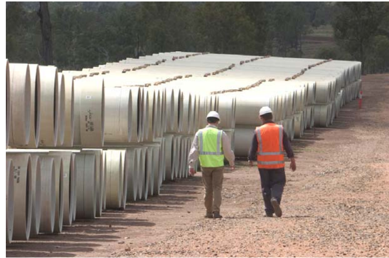
Pipe Stockpile near Caboonbah May 07
