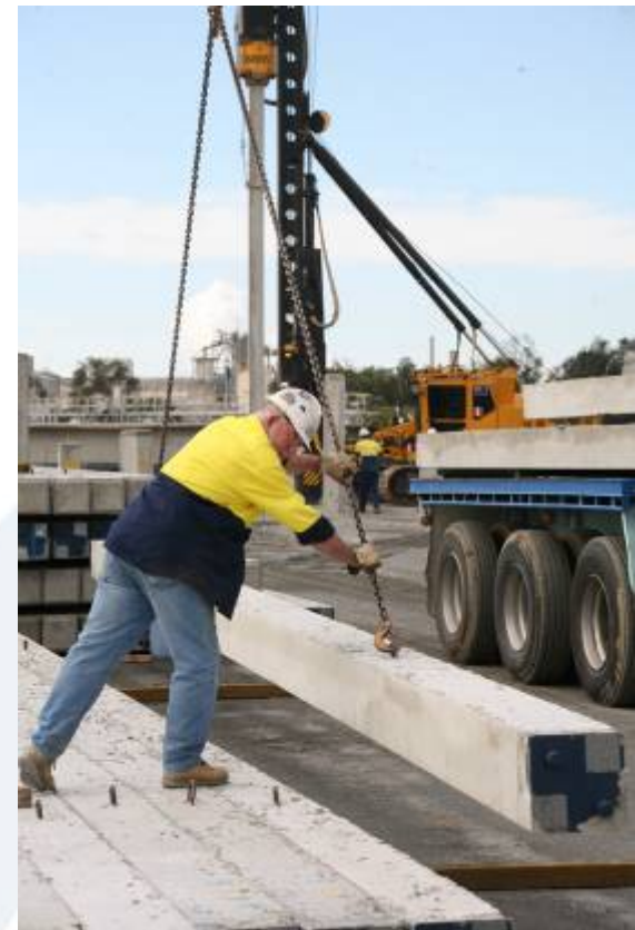
Piling Works at Gibson Island May 07
