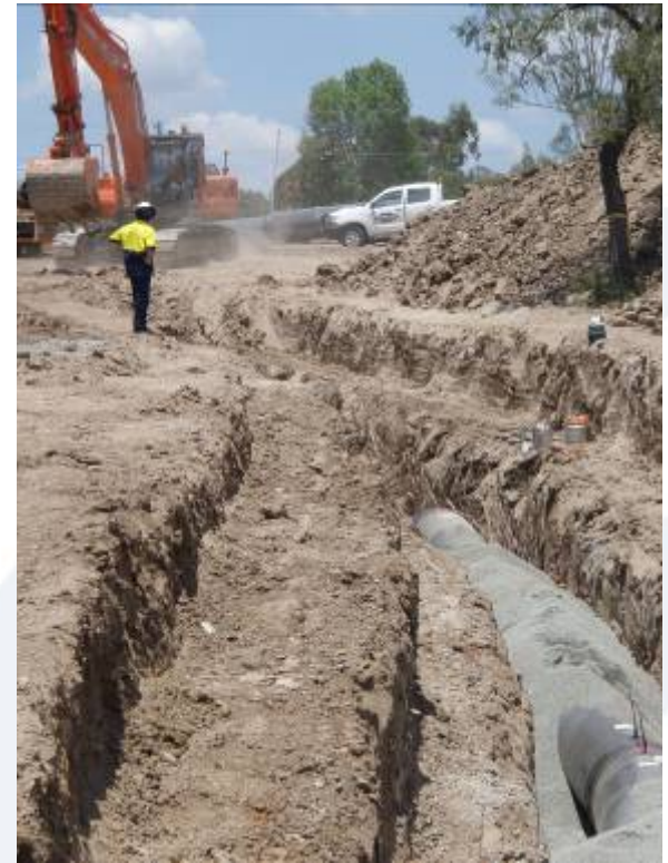
WCRWP Pipe laying at Bundamba, February 07
