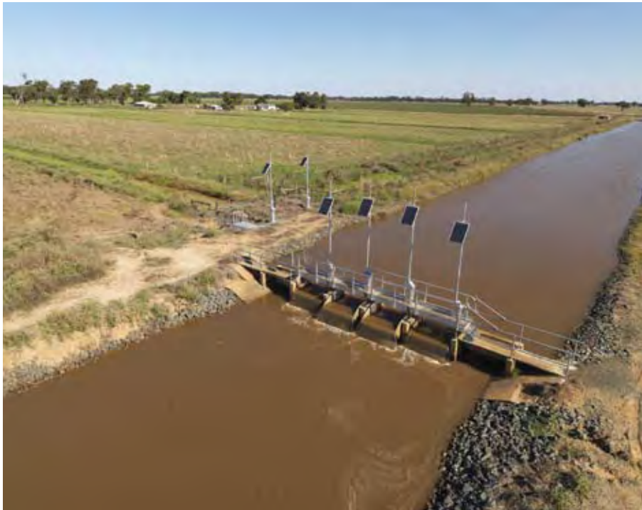
FIGURE 3 REMOTELY CONTROLLED, AUTOMATED FLUMEGATE™ REGULATORS IN VICTORIA
